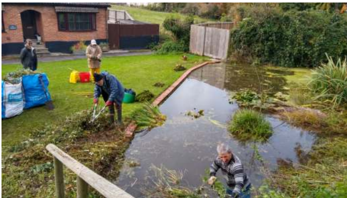
Work well under way
