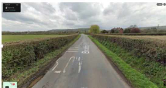
Imagery of Bratton Road in March 2024 via Google Maps
